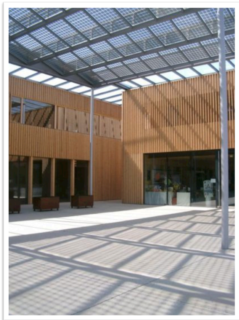
Municipality centre Ludesch/Austria – 2006 120 módulos – 350 m 2 - 19,08 kWp
