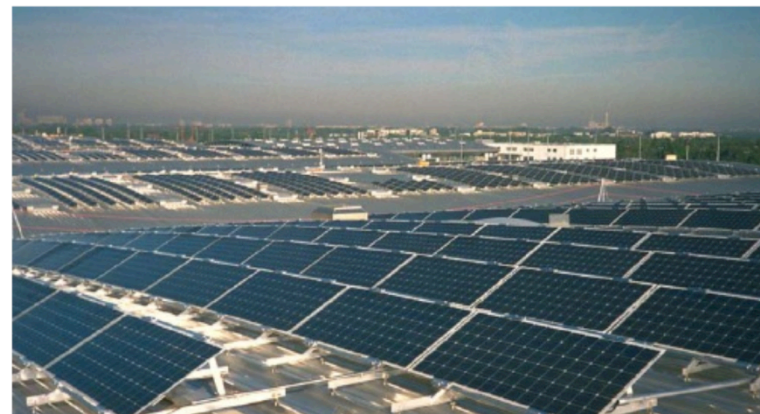
Munich Trade Fair Centre, 2001- 1 MWp
